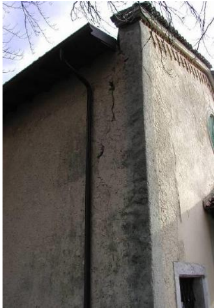
Overturning of façade
