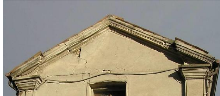
Overturning of upper part of façade
