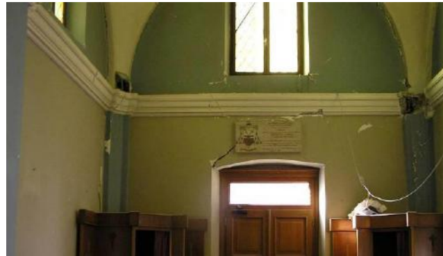
In-plane mechanisms on façade
