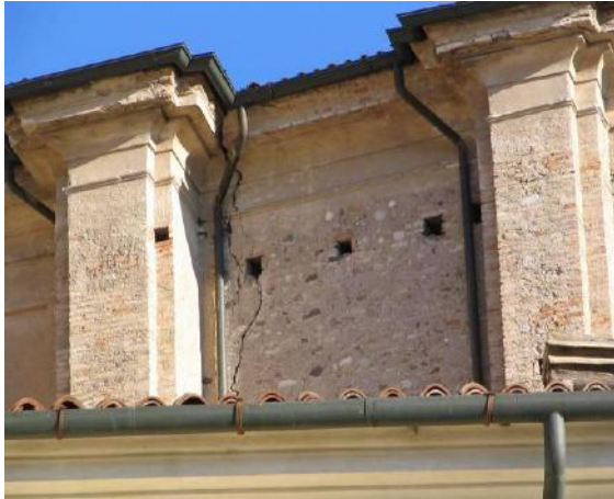
Interaction due to plan-elevation irregularities
