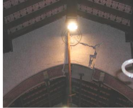
Kinematic mechanism of triumphal arch
