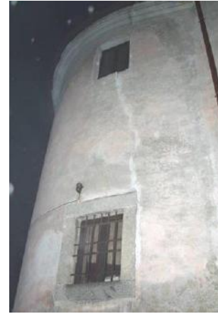
Overturning of apse
