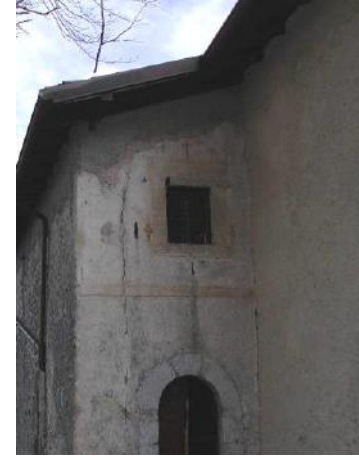
Overturning of side chapels
