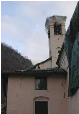
Interaction due to plan-elevation irregularities
