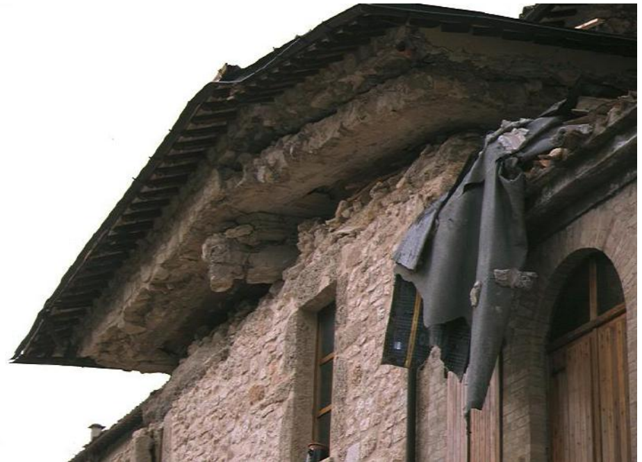
Rigid sliding of roof
