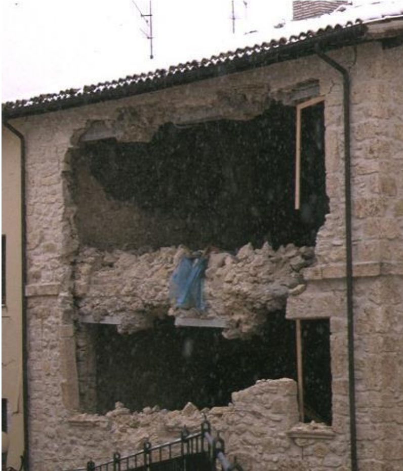
Expulsion of the façade
