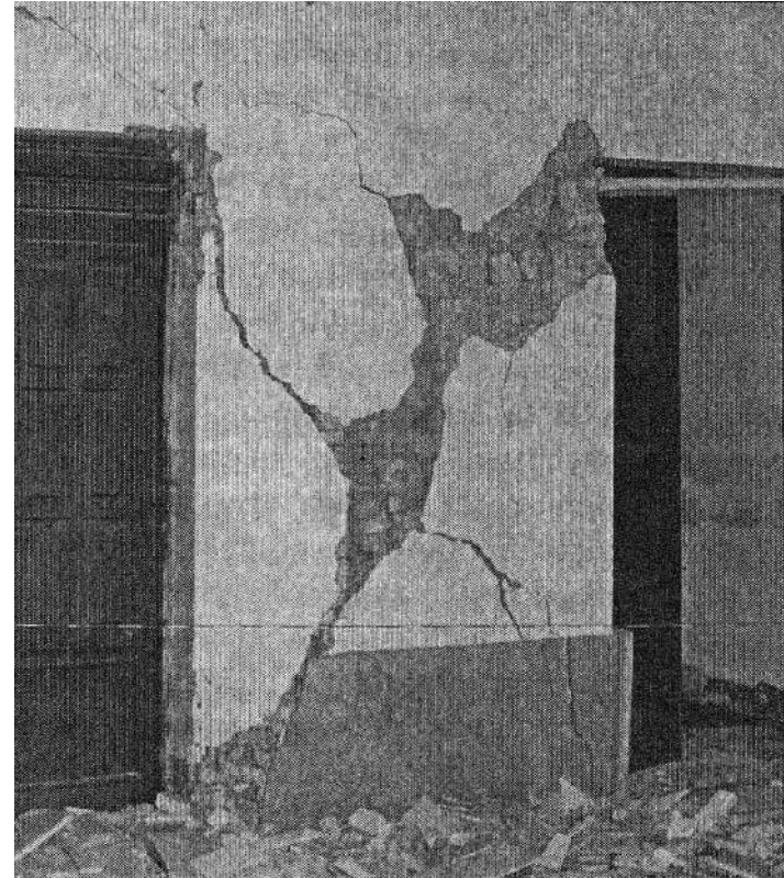
Flexure (and shear) in a slender wall
