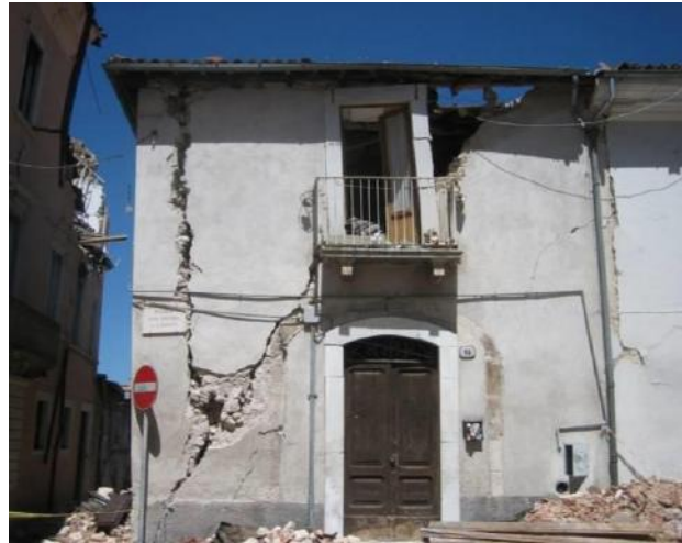
ABSENCE OF TIES
