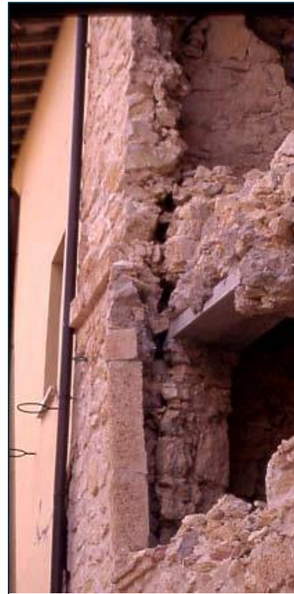
Collapse of a repaired walls
