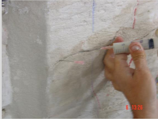
Sealing cracks
