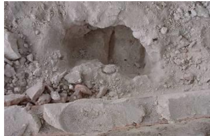
Ribs visual inspection
