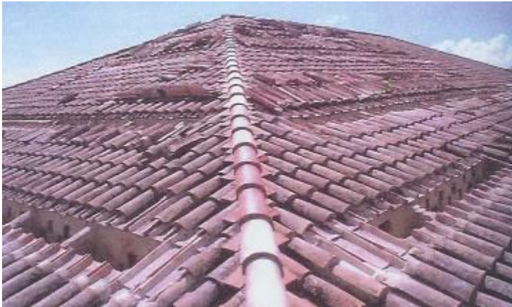
Tiles removal for visual inspection
