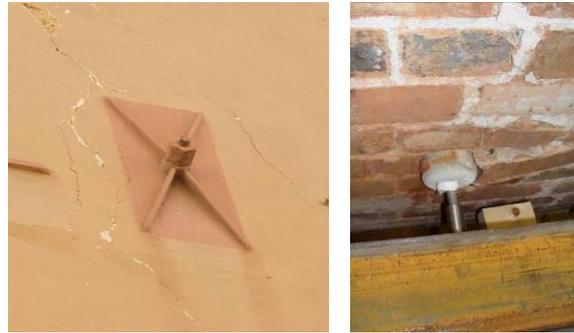
E.g. Standard anchor in masonry substratum
