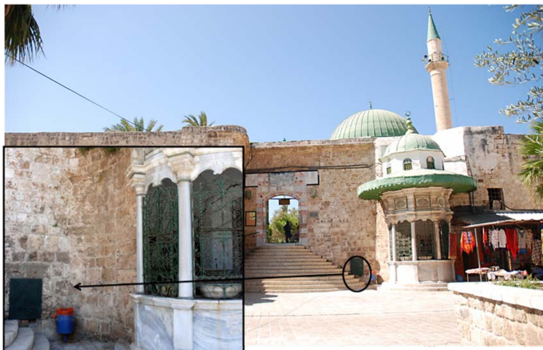
Fig. 3: Main gate to the mosque (north wall) where the grate indicates the end of the cisterns as well as the emergency exit. (Photo: B. Radojewski)
