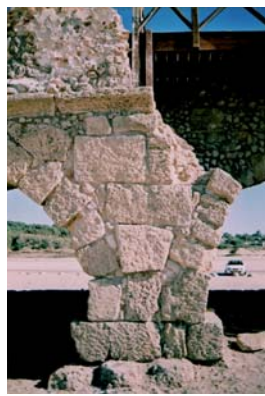
Figure 34. Joint Fill and Stabilization of Collapse of B. (IAA)
