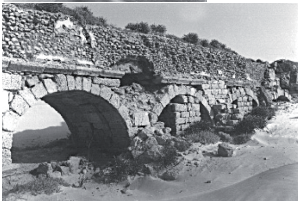
Figure 28. Buttressing of Western Aqueduct. (IAA)
