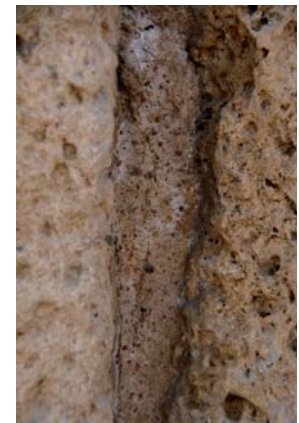
Figure 38. Salt Crystallization. Detail.
