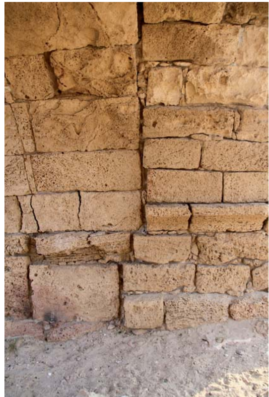
Figure 29. B Leaning on A, Causing Cracks. (David Zell, IAA)
