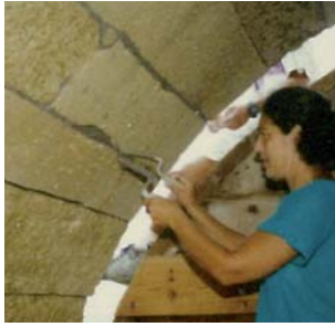
Figure 53. Joint Filling Using Spatula and Trowel. (IAA)
