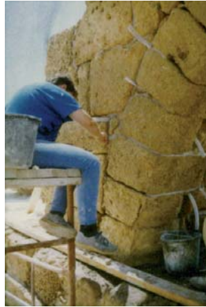
Figure 54. Joint Filling Around Grouting Pipes. (IAA)
