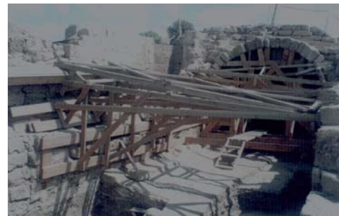
Figure 43. Supports on Vault 1. Facing Northeast. (IAA)
