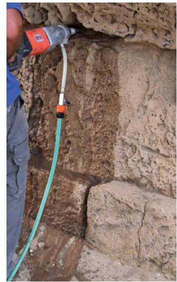
Figure 87. Clear Water During Wet Drilling.
