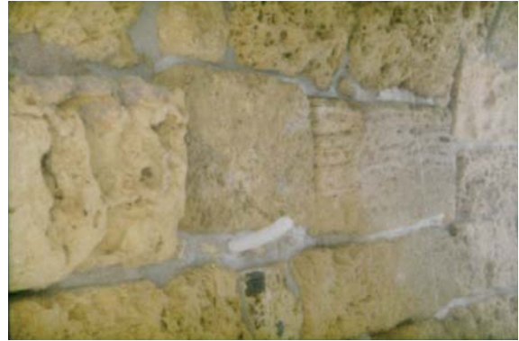
Figure 55. Joint Filling. Finished. (IAA)
