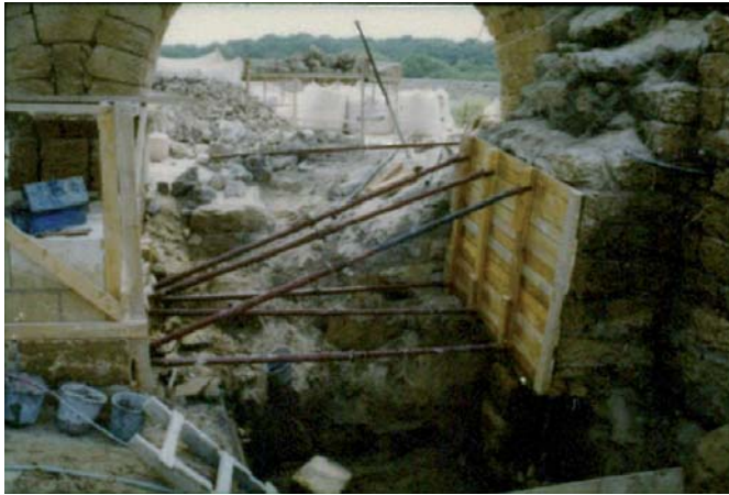
Figure 46. Supporting Wall on Aqueduct. (IAA)
