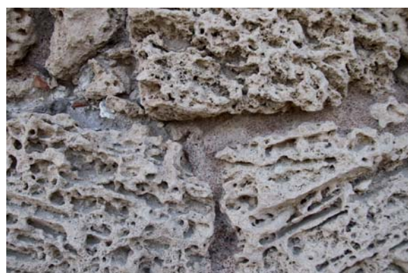
Figure 40. Deterioration of Mortar and Sandstone. Detail.
