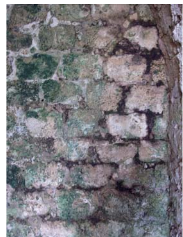
Figure 14. Biological Growth and Salt Crystallization. Vault 1. East Wall.
