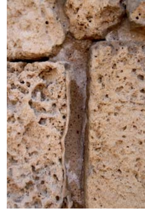
Figure 37. Salt Crystallization.
