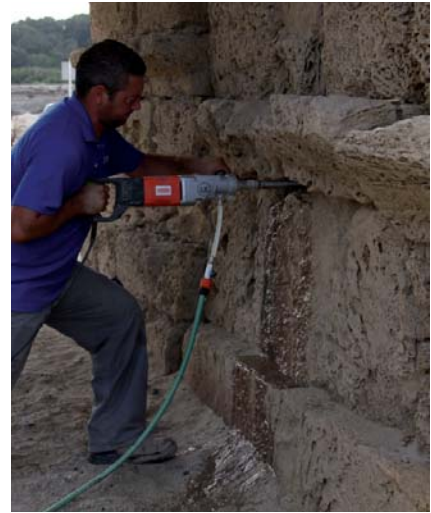
Figure 82. Wet Drilling.
