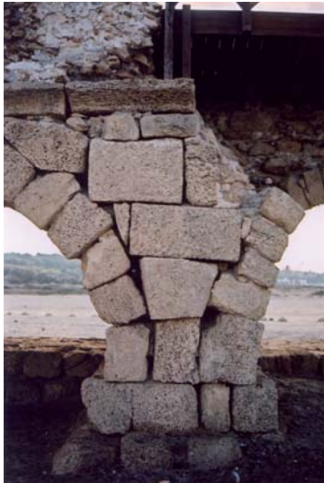
Figure 67. Before Joint Filling. 1991-93. (IAA)
