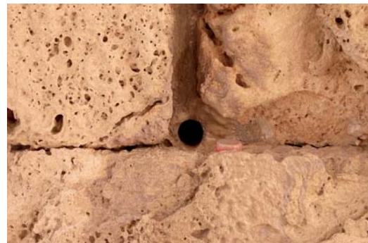
Figure 79. Placement of Core Drill.
