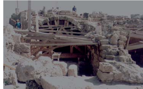
Figure 42. Supports on Vault 1. Facing East. (IAA)
