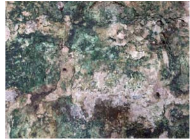
Figure 15. Biological Growth and Salt Crystallization. Detail. Vault 1. East Wall.
