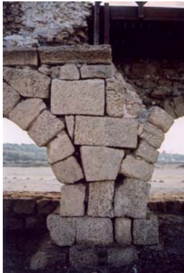
Figure 33. Missing Mortar and Collapse of B. (IAA)
