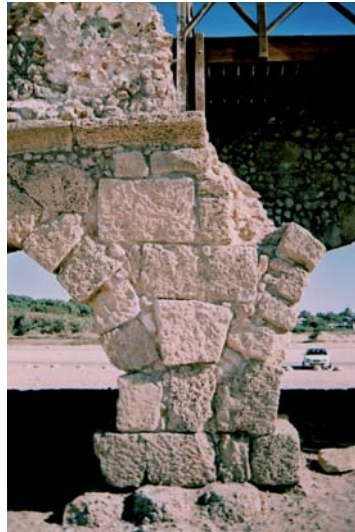
Figure 68. After Joint Filling. 1991-93. (IAA)
