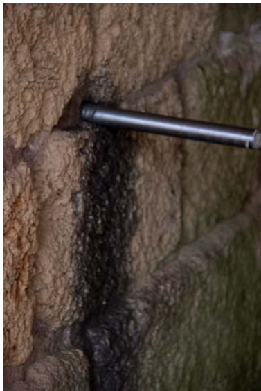
Figure 85. Black Water During Wet Drilling.
