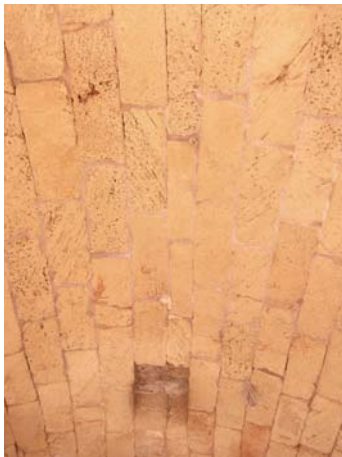
Figure 61. Joint Fill. Vault 1, Ceiling.
