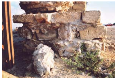
Figure 31. Exposed Rubble Fill and Foundation. (IAA)
