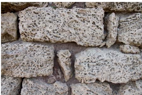
Figure 39. Deterioration of Mortar and Sandstone.
