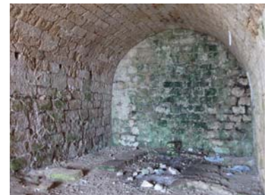
Figure 16. Biological Growth and Salt Crystallization. Overview. Vault 1. East Wall.
