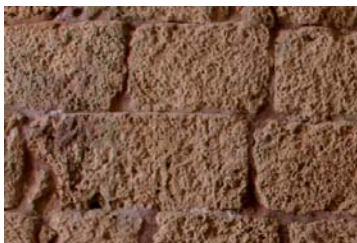
Fig 62. Joint Fill. Vault 1, North Wall (Covered).
