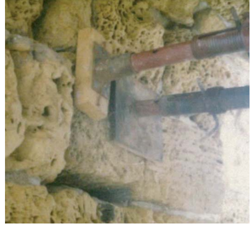
Figure 47. Metal Supports with Wooden Buffer on Aqueduct. Detail. (IAA)
