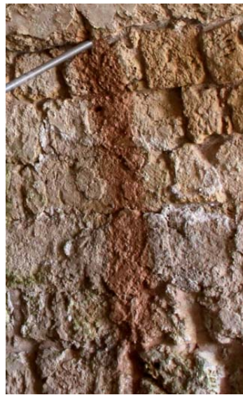
Figure 86. Brown-Red Water During Wet Drilling.
