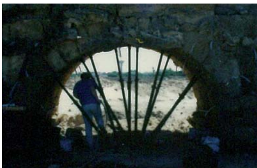
Figure 44. Metal Supports on Aqueduct. (IAA)
