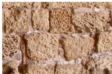
Fig 63. Joint Fill. Vault 1, South Wall (Covered).
