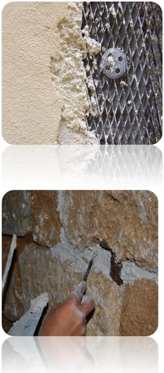
The mortar composition for wall coating is mainly based on lime and crushedstone.
