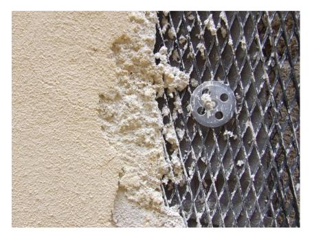
Final Results taken out from the system: so far the plaster and the mortar hold steady in external walls. Regarding the interior walls, the system doesn't seem efficient. Moisture problems haven't been 100% solved inside the buildings, therefore the plaster starts to crack and fall.
