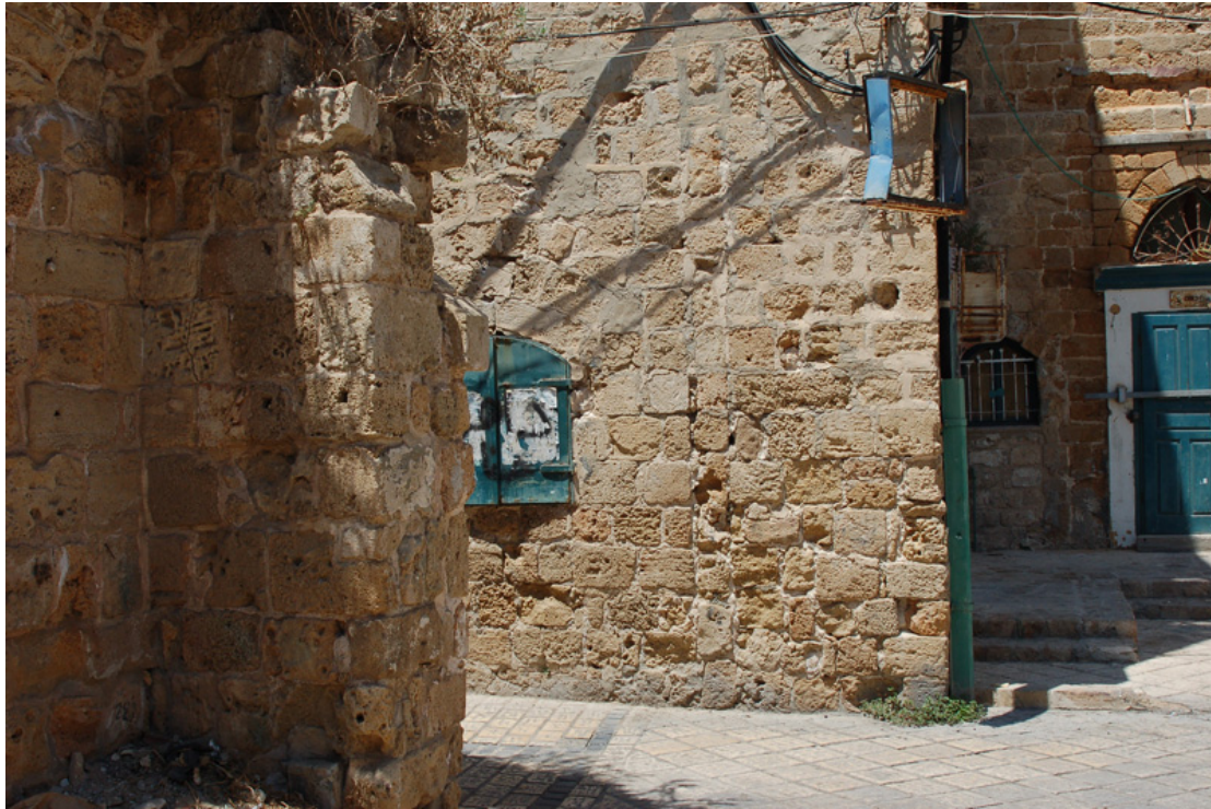
The southern façade of the west wing shows a vertical arrangement of stones and joints, revealing the outline of the past wing since removed.
