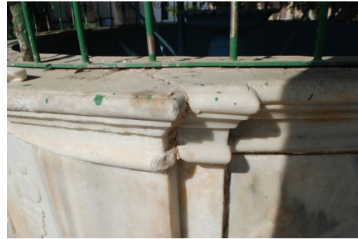
Interior well, constructed entirely of white marble, incorporates pilasters and carved detailing to identify each individual ablutions unit.
