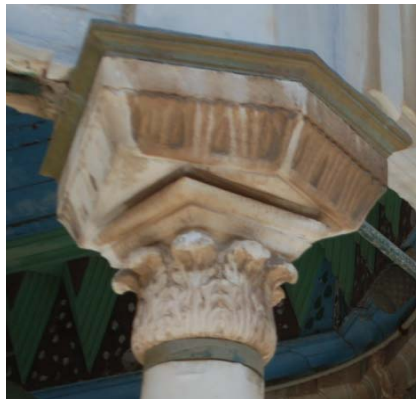
Marble beams and cornice above columns act to add structural support. Cantilevered octagonal roof extends beyond the beams.
