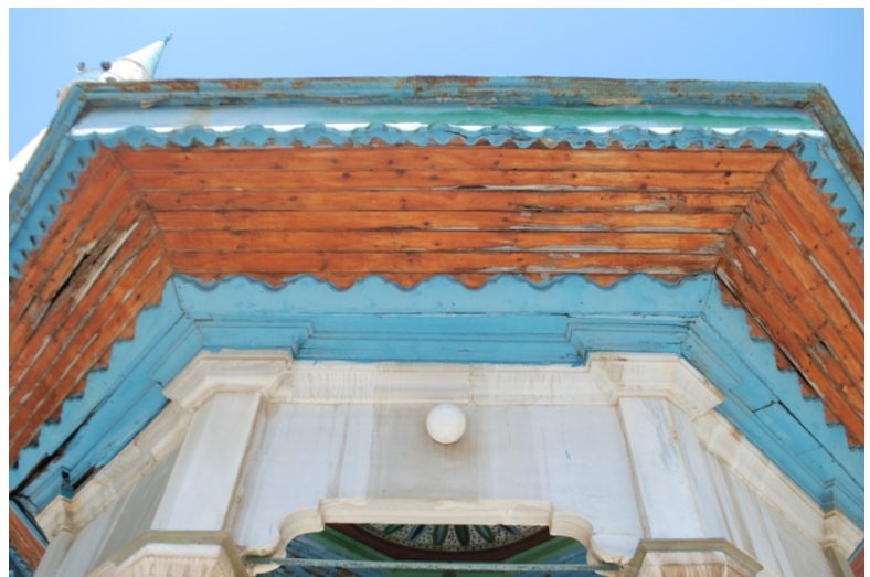
Marble beams and cornice above columns act to add structural support. Cantilevered octagonal roof extends beyond the beams.
