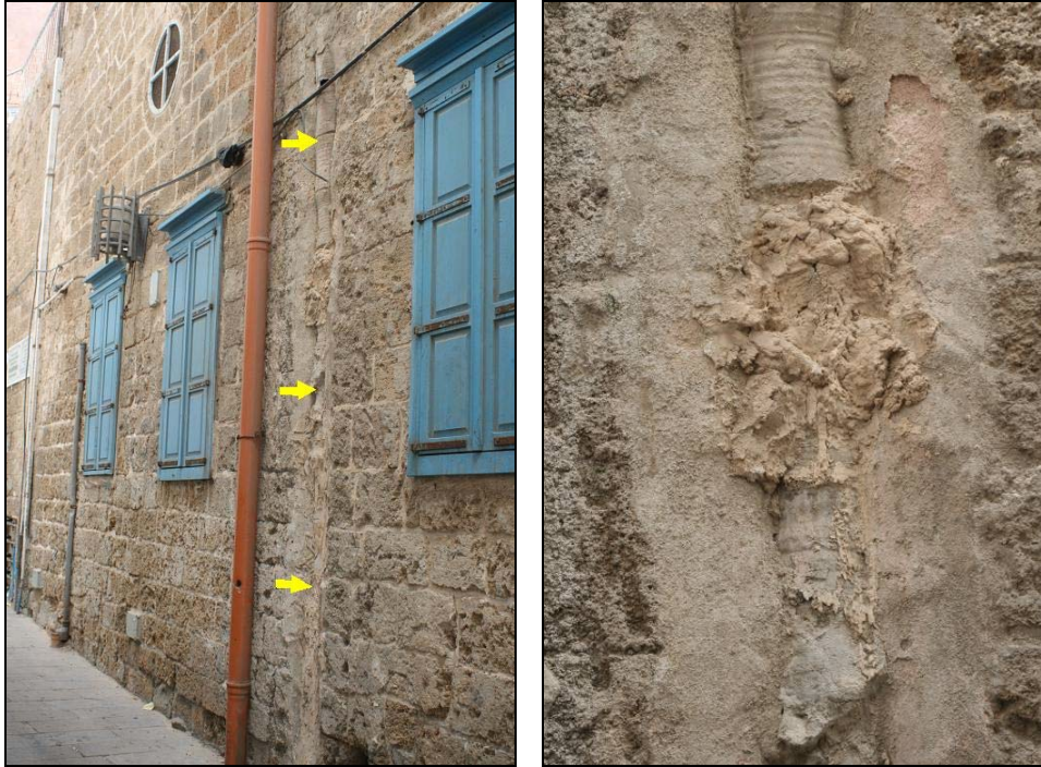
Fig. 2 & 3 (detail). Ottoman cistern pipes embedded in wall.
