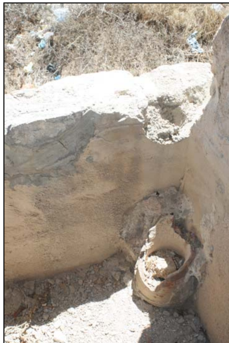
Figs. 30 & 31. Stone pipe through which water entered the basin of the tower and clay pipe through which it exited.
