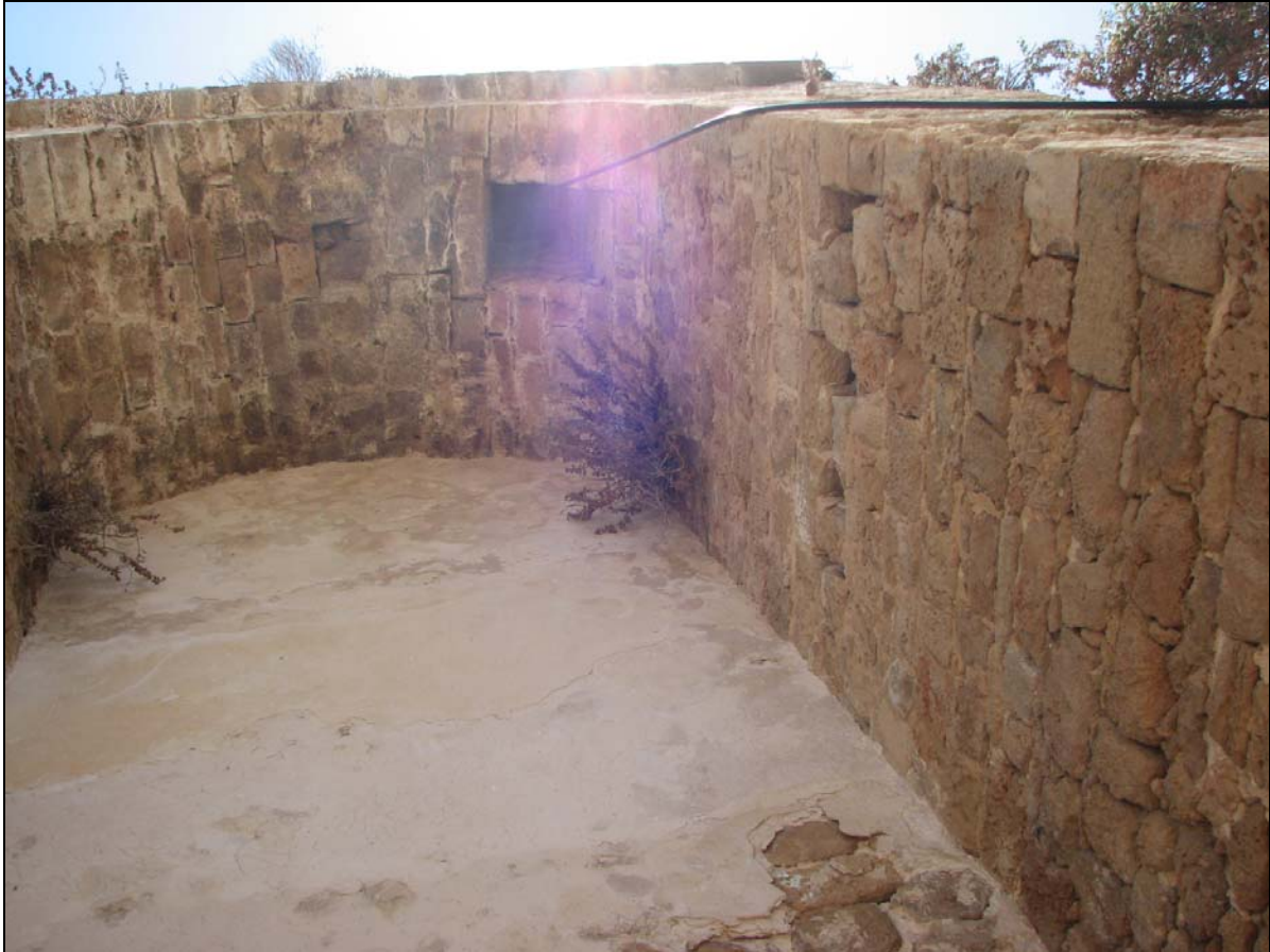
Fig. 20. Hole in arch through which the water in the tub below could be tapped.
