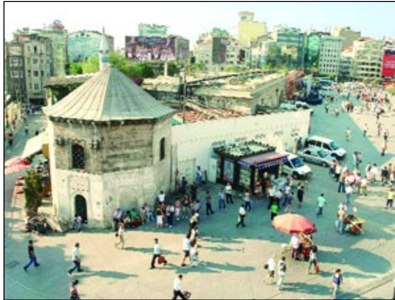
Fig. 50. Distribution tank ( maksem ) in Istanbul, Turkey.
