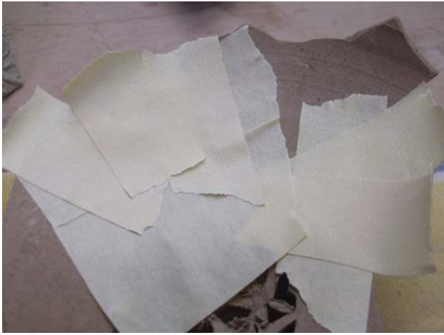
Above: Img. 38 Masking tape applied in a criss cross fashion to provide adequate support for the plaster fill
