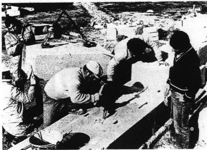
Figure 19. Metapontum, theatre. Natural stone used in rebuilding the outer wall, with strict adherence to ancient technique of working.
