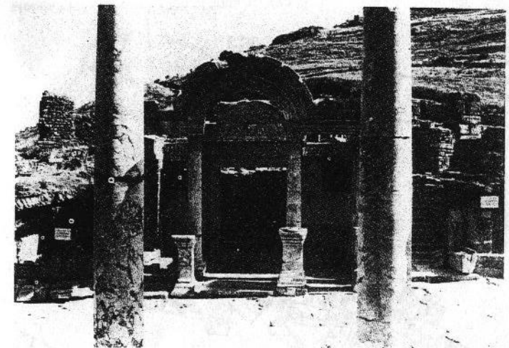
Figure 5. Ephesus, Temple of Hadrian. Anastylosis carried out almost exclusively with original building elements.
